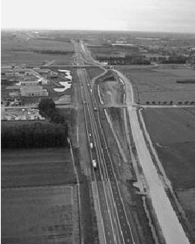
Figure 3-4. Betuweroute Parallel to a Roadway.
