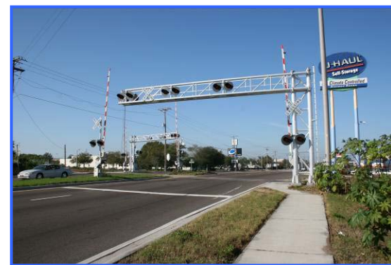
Port Tampa Spur grade crossing at Gandy Boulevard near the Lee Roy Selmon Expressway.
