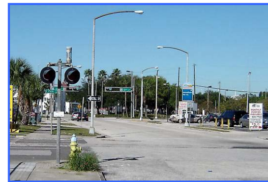
Ungated signalized grade crossing at Jefferson and Polk Streets in downtown Tampa.
