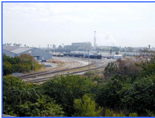
CSX BIDS Transflo Terminal located south of the Lee Roy Selmon Expressway.
