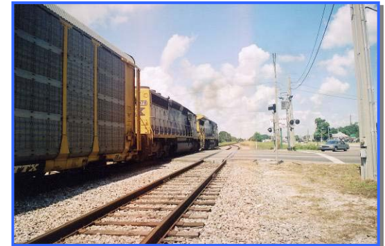
Lakeland Subdivision mainline grade crossing at US 92 and Park Boulevard, Plant City.
